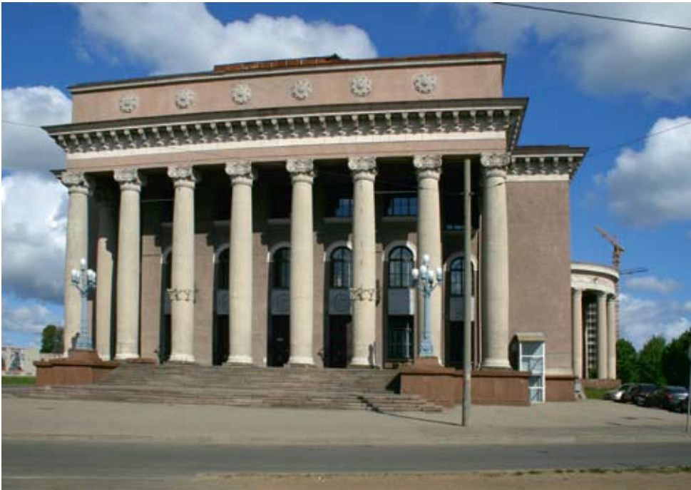
8. VEF Palace of Culture. Photo by Aivars Holms, 2008. Monument Documentation Centre of the State Inspection for Heritage Protection, Republic of Latvia.
